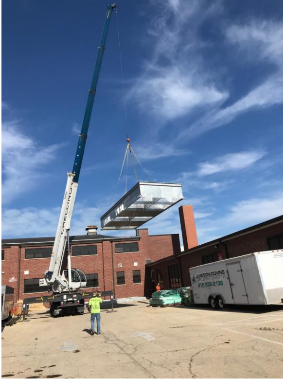
RTU Curb Installation
